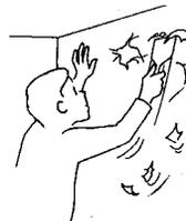
2. **DO NOT** sandblast or waterblast lead-based paint on the outside of your home. You do not want the paint chips to end up all over your yard or the neighbor's yard. Sandblasting and waterblasting is safe **ONLY** if you have a special machine that will catch the paint chips.
